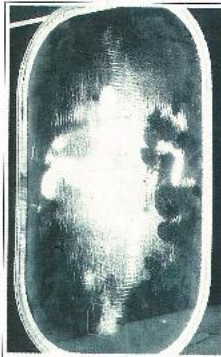
Line crazing: concentrated in the centre of the window.
